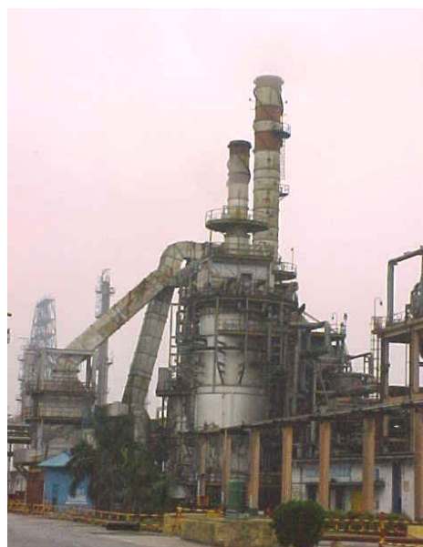
AVU-I Furnace Stack
