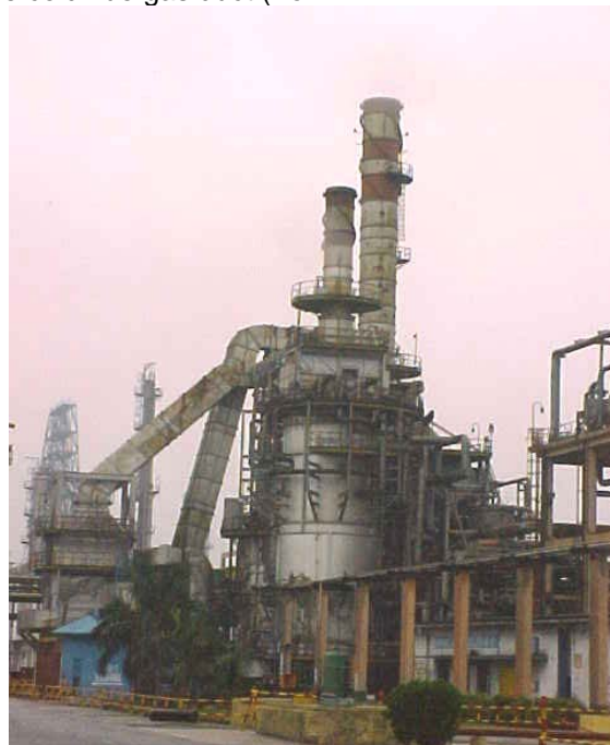
AVU-I Furnace Stack
