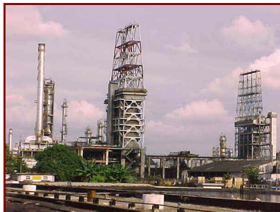
Delayed Coker Units
