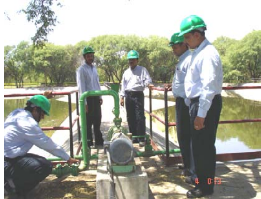
INSTALLATION OF PUMP TO UTILIZE STORM WATER FOR HORTICULTURE
