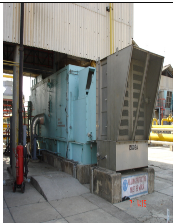
RR Allison Gas turbine compressor
