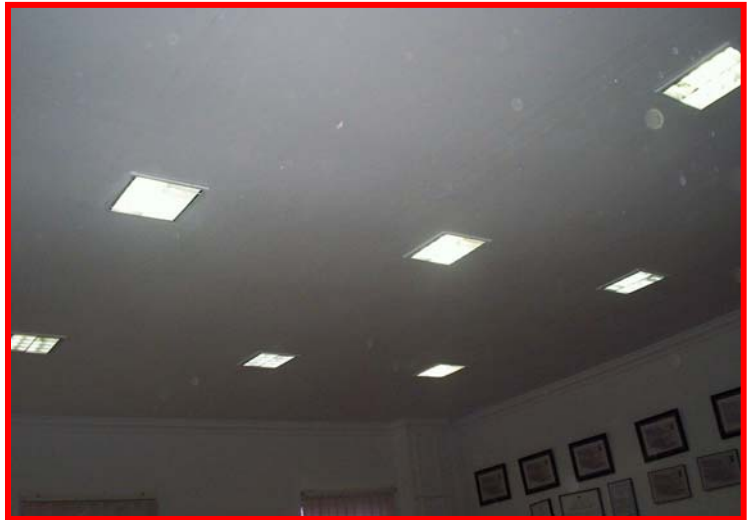
View of Energy Efficient CFL Installation
