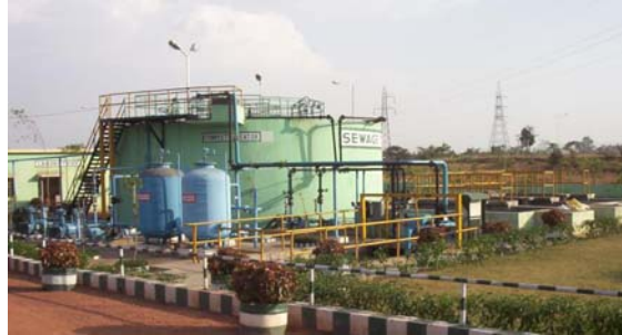
SEWAGE TREATMENT PLANT-II
