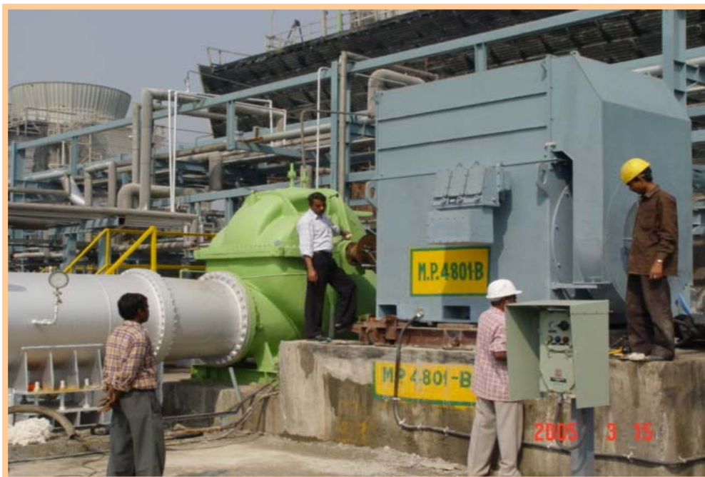
Photograph of LTS Guard Reactor installed in Ammonia-II
