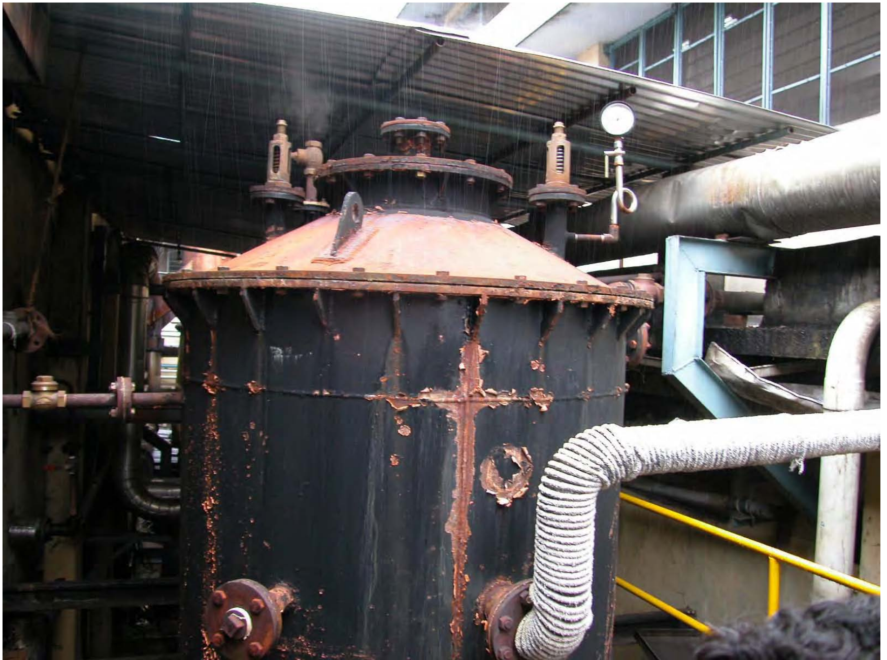
Condensate Recovery Tank
