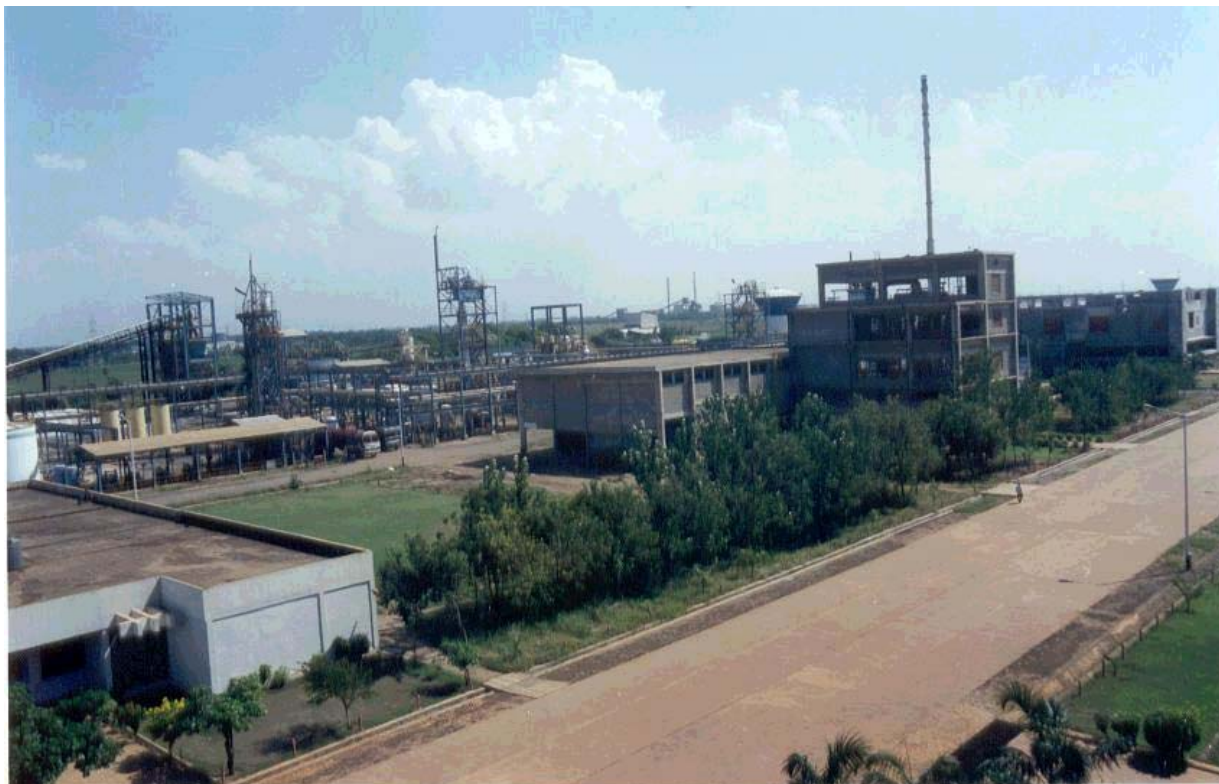
(An overview of plant)
