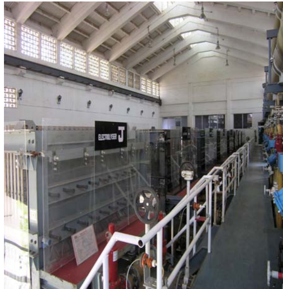
ADDITION OF 9 TH ELECTROLYSER
