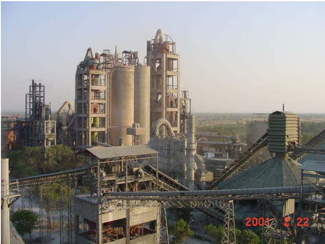
A VIEW OF THE PLANT
