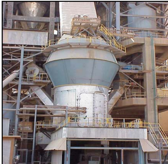
Fig : Vertical Roller Mill at Gujarat Cement Works at Kovaya
