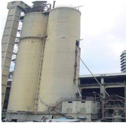
Dry Fly ash Storage
