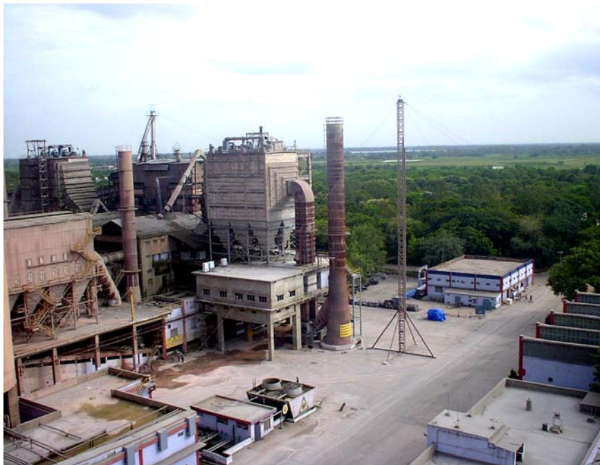
Electro Static Precipitator installed at clinker cooler
