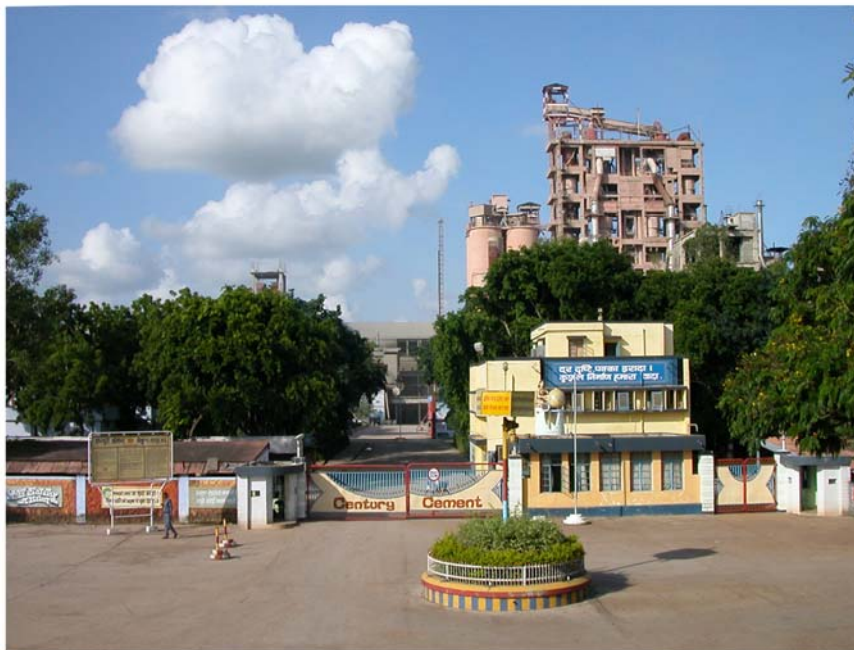
A view of the Plant
