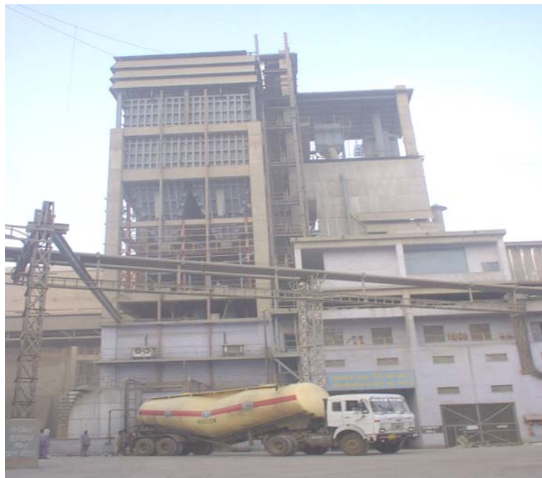
Dry Fly Ash Handling System
