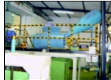
Foam recycling plant
