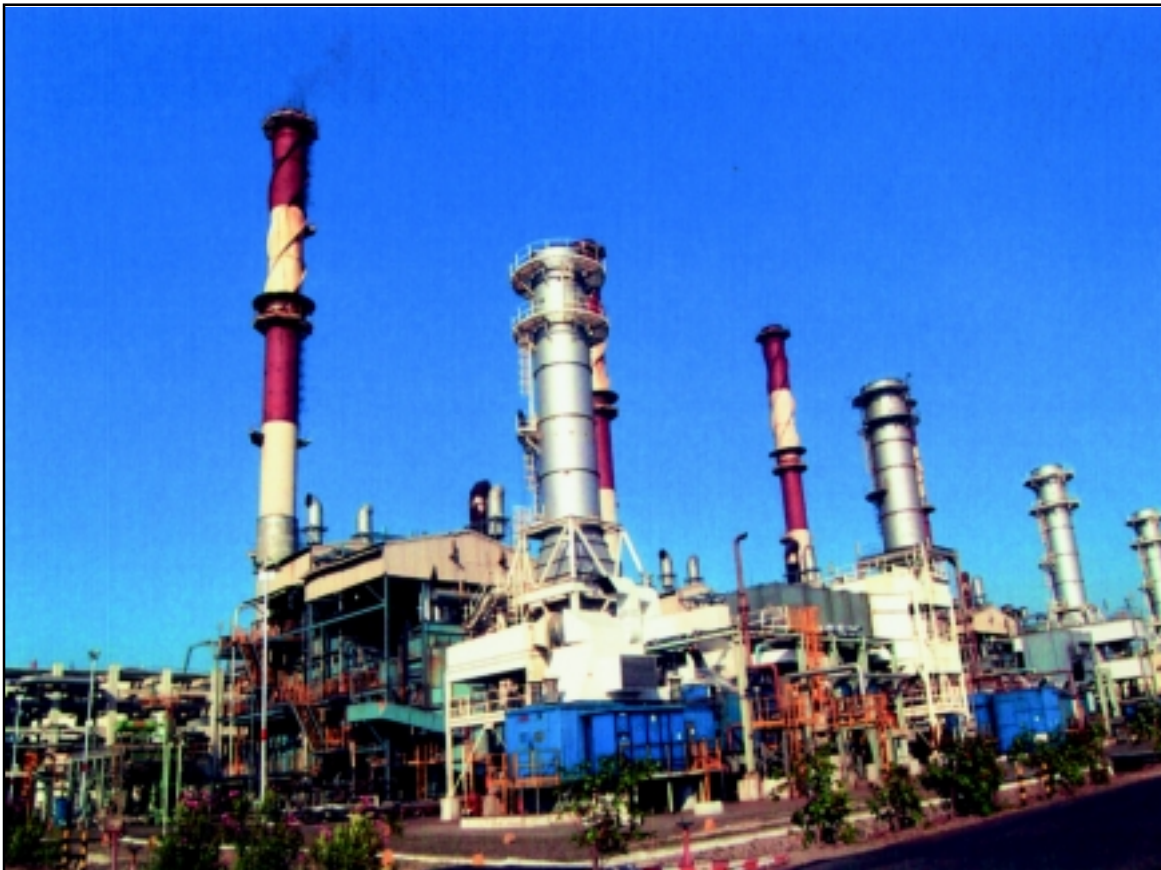
Highly Efficient Co-generation Captive Power Plant
