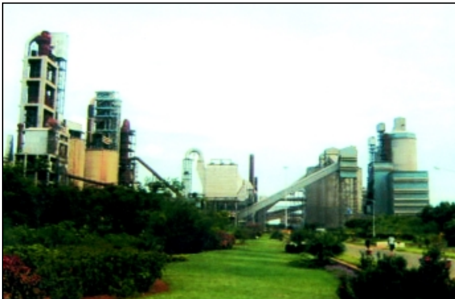
An overview of the Alathiyur Plant
