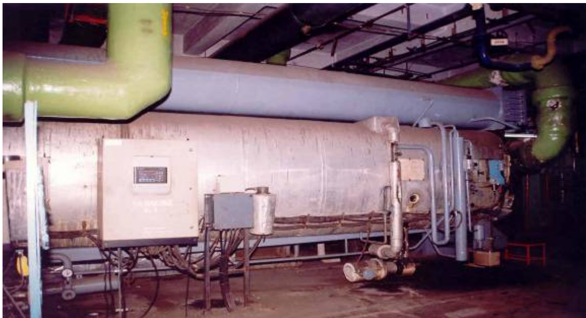
SINGLE EFFECT VAPOUR ABSORPTION & REFRIGERATION MACHINE
