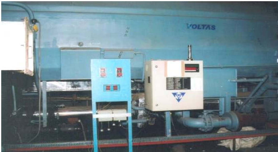
DOUBLE EFFECT VAPOUR ABSORPTION & REFRIGERATION MACHINE
