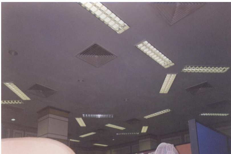
Light & VFD upgrades
