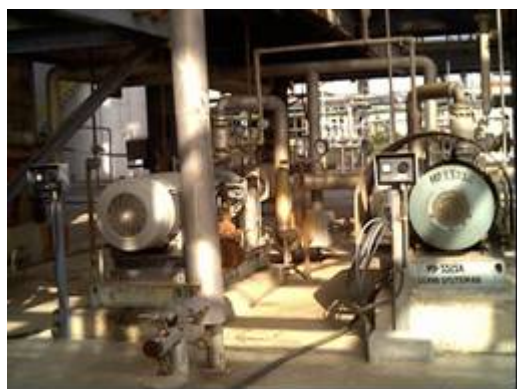
P-3323B Turbine Replaced with Motor
