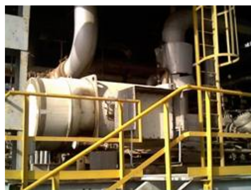
Running of Standby GV Solution Pump Motor And stopping of one condensing turbine.
