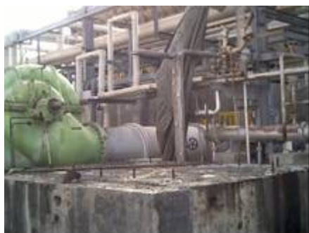
Replacement of Condensing Turbine in Urea-II Cooling Tower
