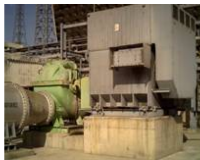
Running of Standby motor in Amm-II CT and stopping of One condensing turbine
