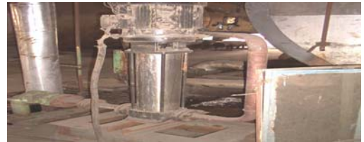
Reduction in load from 18.5 KW to 15 KW
