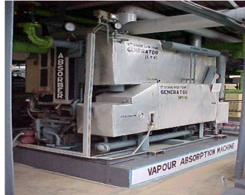
VAPOUR ABSORPTION SYSTEM
