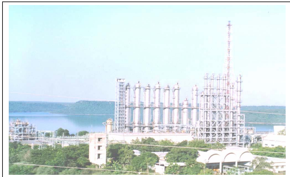
AN OVERVIEW OF HEAVY WATER PLANT,KOTA
