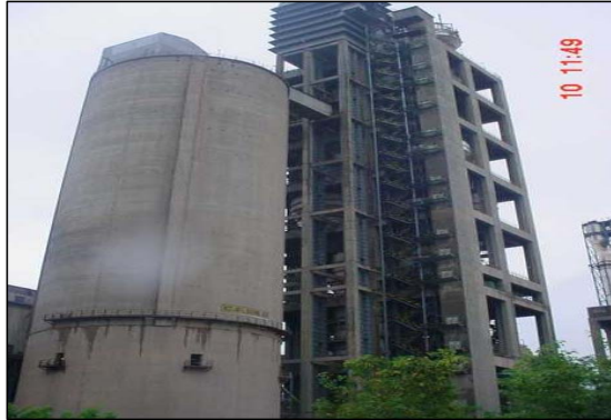
RABH ,MAIN CHIMNEY & PRE-HEATER
