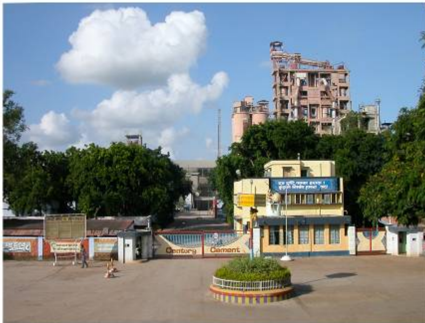
A view of the Plant
