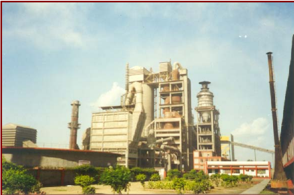
An Overview of "Satna Cement Works" Plant
