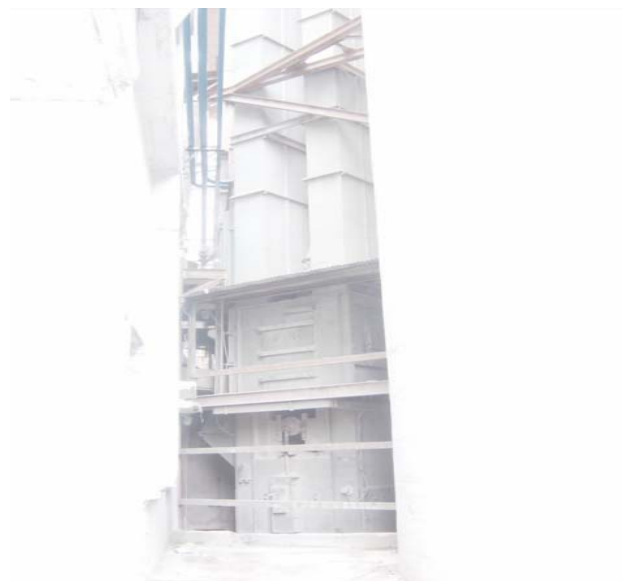
Belt Bucket Elevator In Raw Mill
