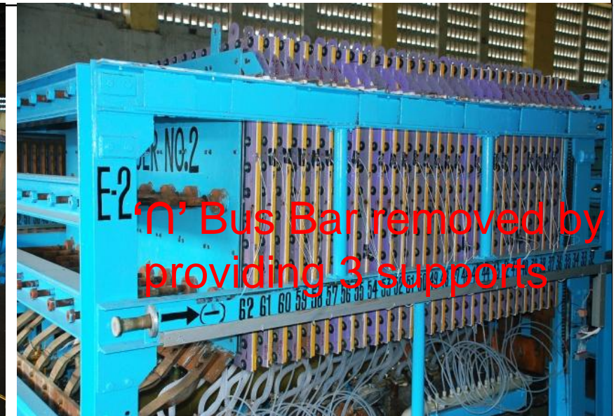
Removal of 'n' bus bar and addition of five more elements
