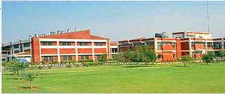
Dharuhera Plant - Haryana Production Started 1985 ←
