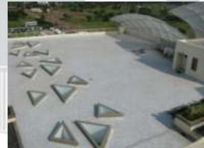
USE OF STYROFOAM AND CHINA MOSAIC FOR TERRACE
