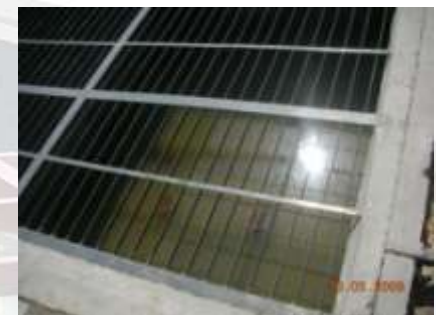
RAINWATER RECHARGE PIT
