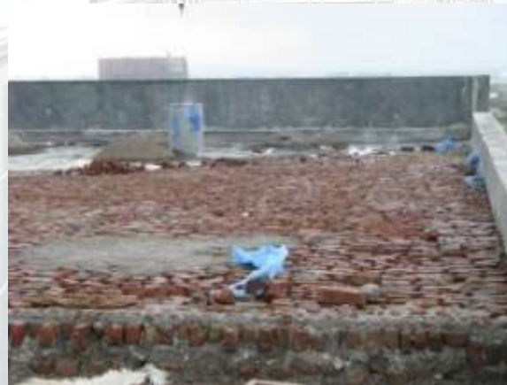
BRICKBATS FOR WATERPROOFING
