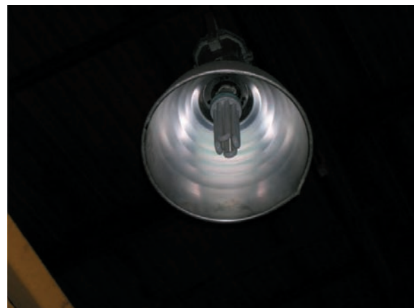
HPMV & HPSV High Bay Fixtures have been retrofitted by suitably modifying with 2 pin porcelain Lamp Holder to suit the 85W/65W CFL Lamps.
