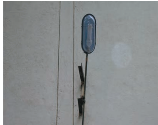
The HPMV and HPSV of 400W and 250W respectively have been replaced along the perimeter or boundary of the Mint premises by 85W/65W/45W CFL fittings.
