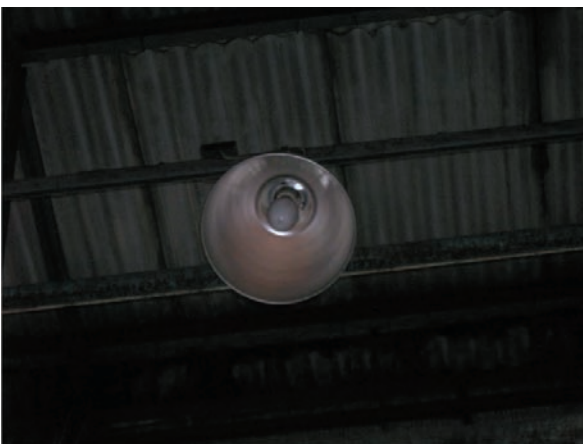
HPMV & HPSV High Bay Fixtures have been retrofitted by suitably modifying with 2 pin porcelain Lamp Holder to suit the 85W/65W CFL Lamps.
