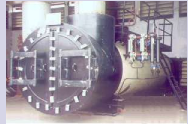
WHRB for 2 X 1 MW gas fired engines
