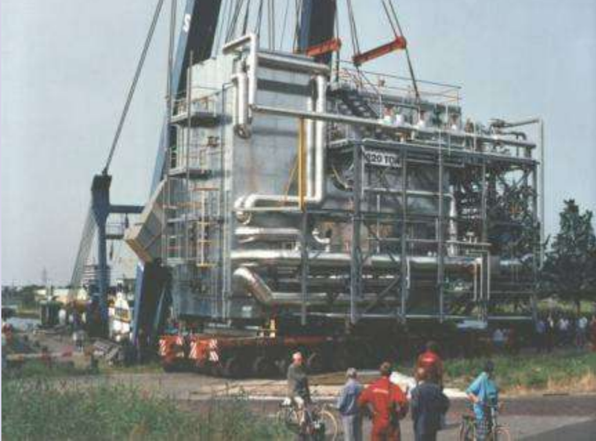
Horizontal compact boiler – 100 TPH
