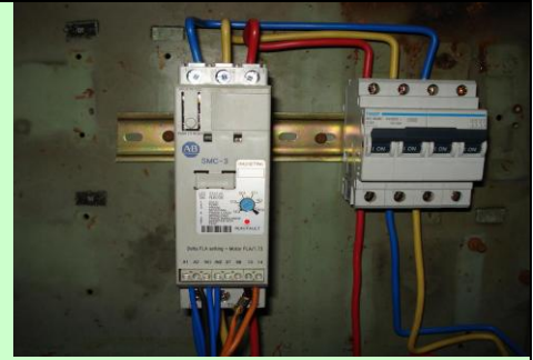
Soft Starter for Vacuum Pump
