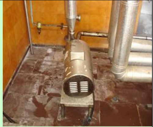
High capacity pump for transferring of milk
