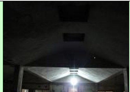
Ghee section without ventilation
