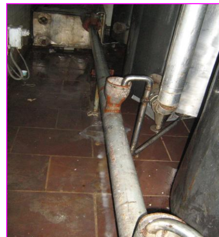
New 4" GI pipe
