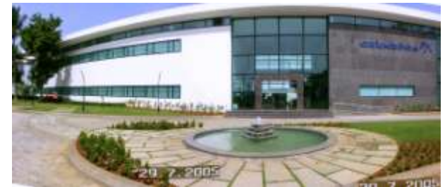
Grundfos Pumps, Chennai Gold Rating
