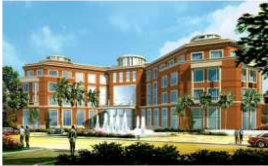
ITC Green Centre, Gurgaon Platinum Rating
