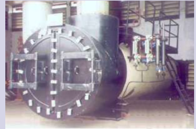
WHRB for 2 X 1 MW gas fired engines
