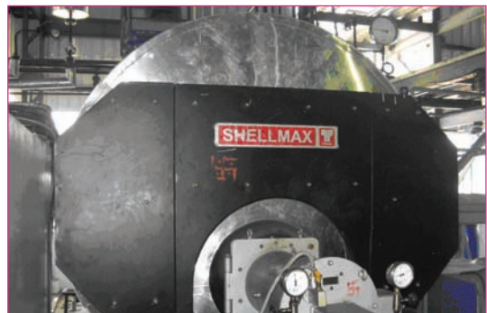
▲ New 5 - Ton IBR Boiler
