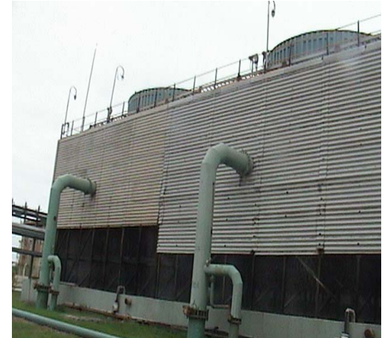
Cooling Tower Revamping
